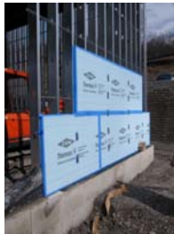
Photo courtesy of Dow Building Solutions
